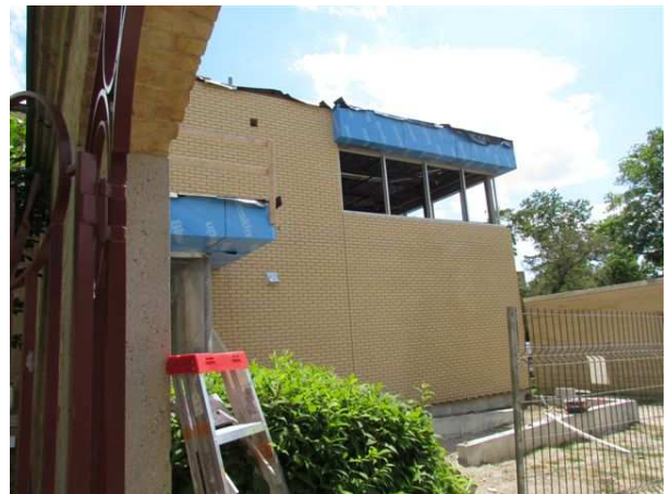
[Construction on the addition to the Governor's House]
