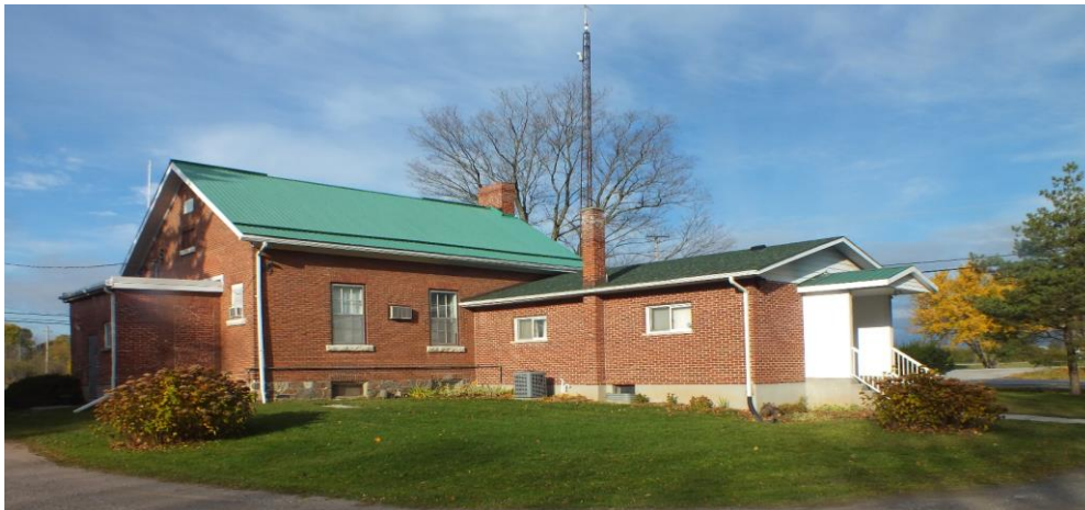
The Trent Valley Archives showing the original school house and the Council Chambers addition.
